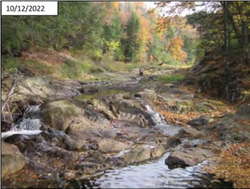
Two Years Post-construction
