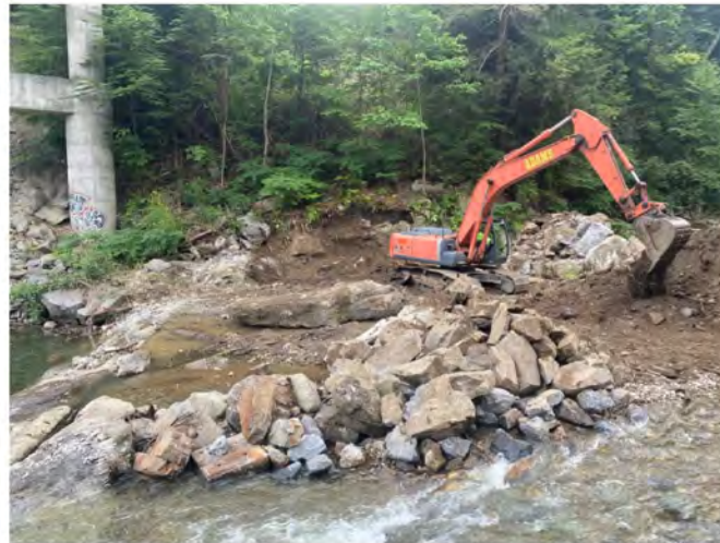
Figure 1: Preparing right bank for stone armor application.
