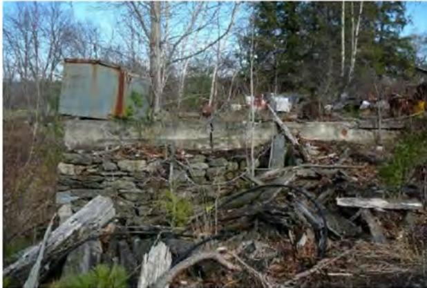
Figure 45. View of the southern side of the mill foundation, looking north. Stone wall may be an extant early mill foundation wall; also note concrete floor on top of stone wall.
