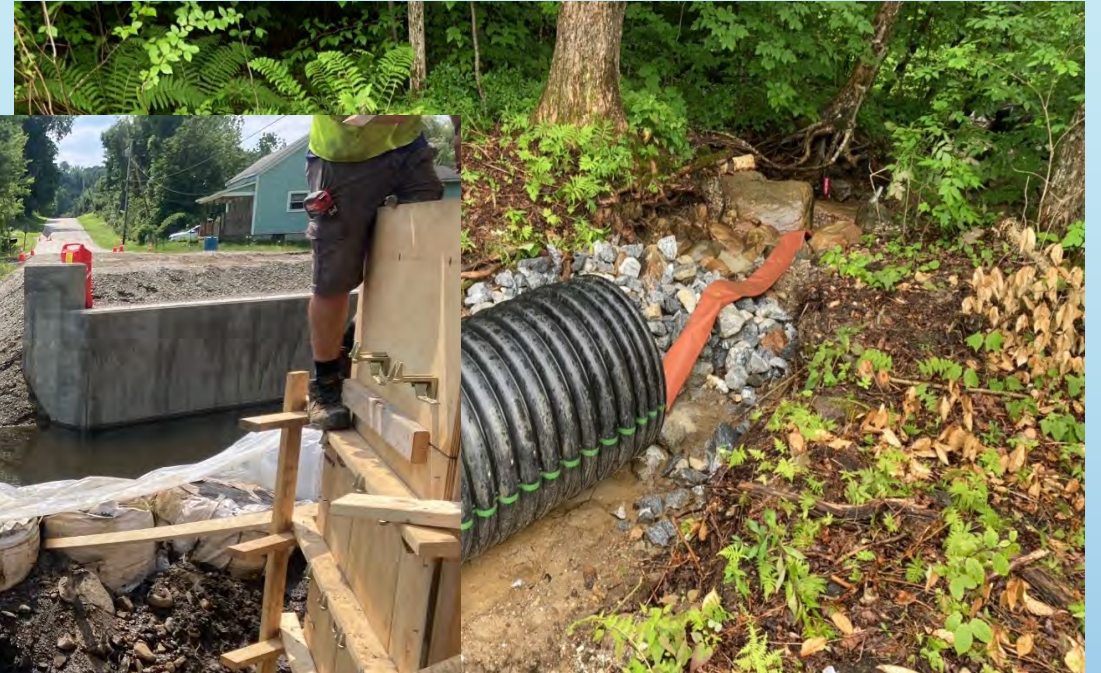
Temporary bypass culvert for stream low flows
