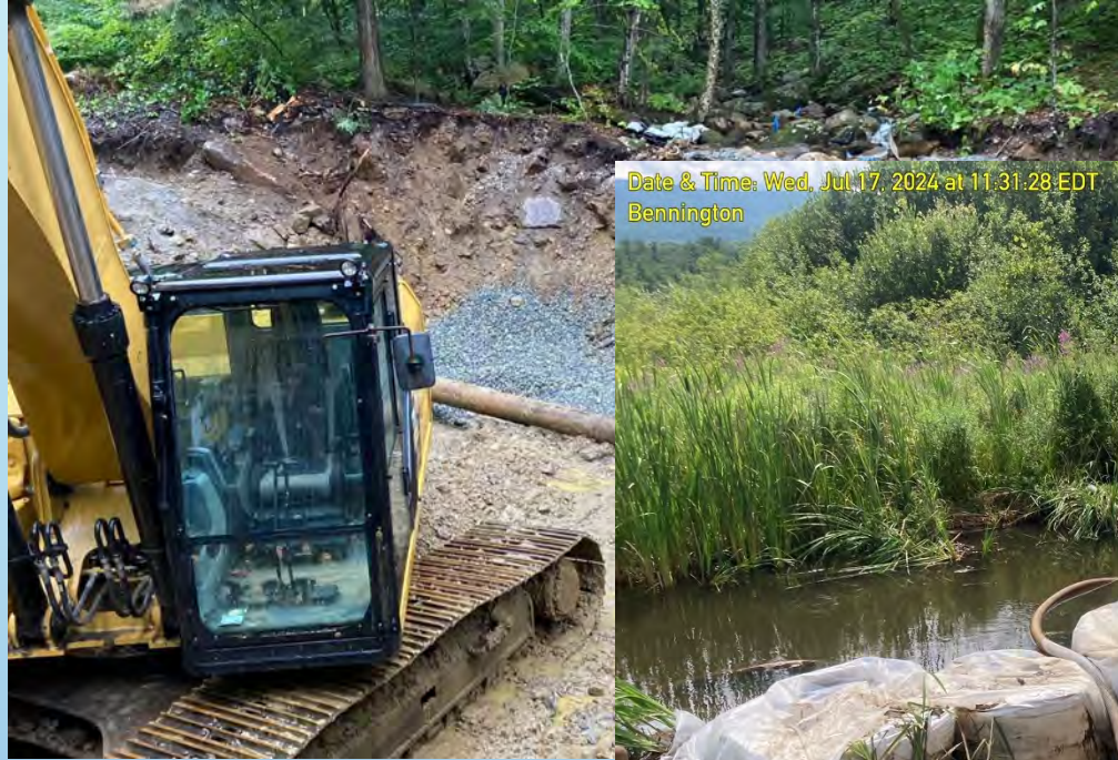
Low point sump with stone for dewatering
