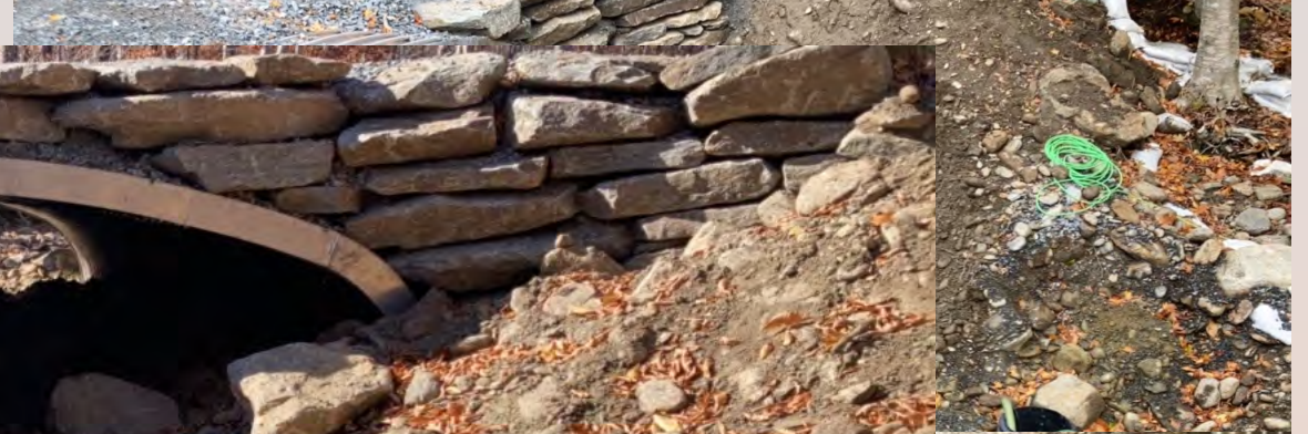
Placement of the mixture larger stone and fines
