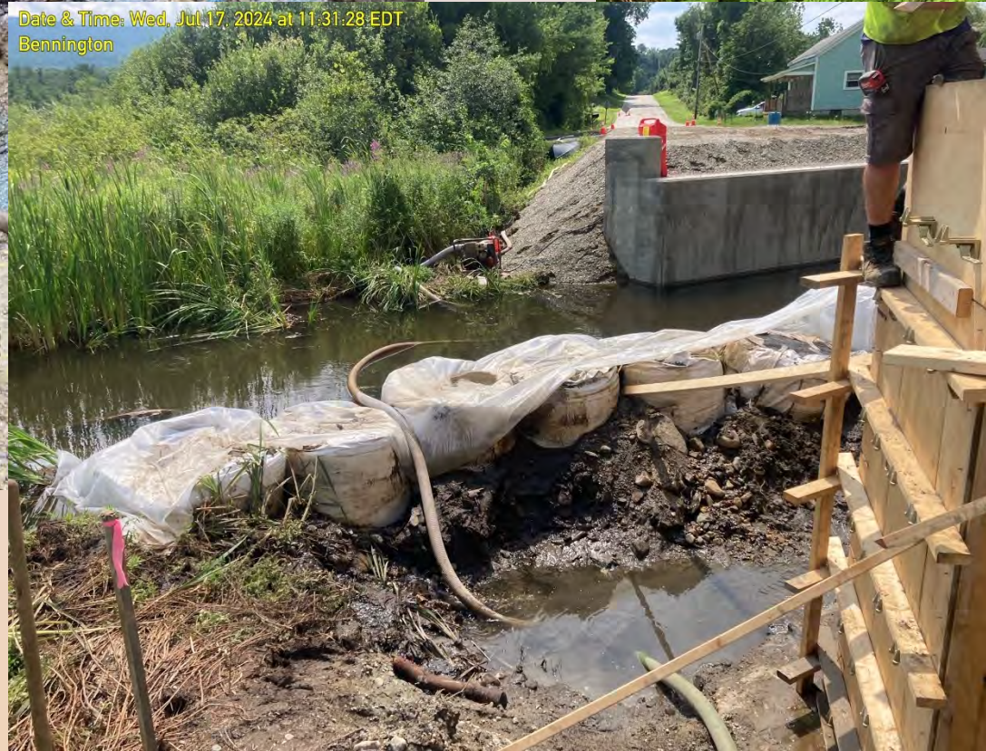
Cofferdam used to isolate the active work area
