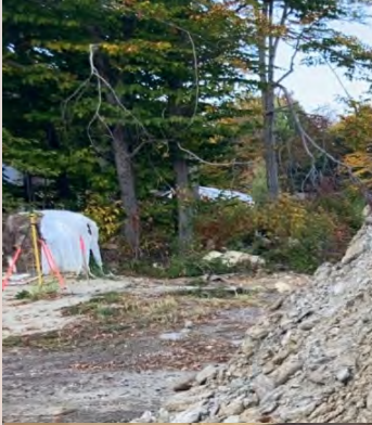
Salvaging the excavated bed material on site
