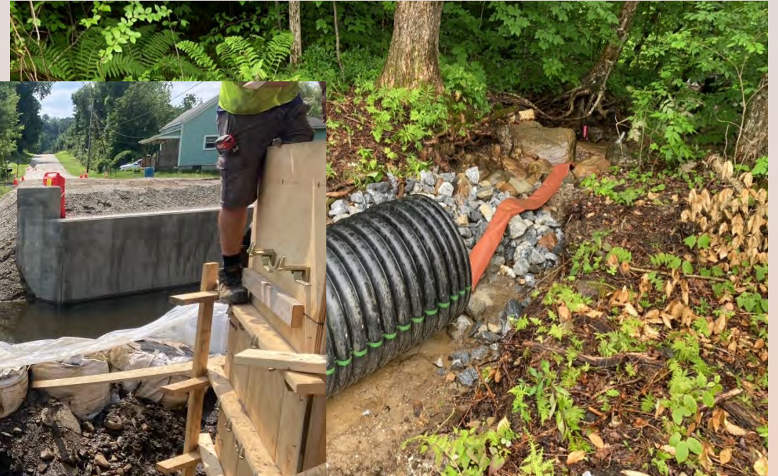
Temporary bypass culvert for stream low flows
