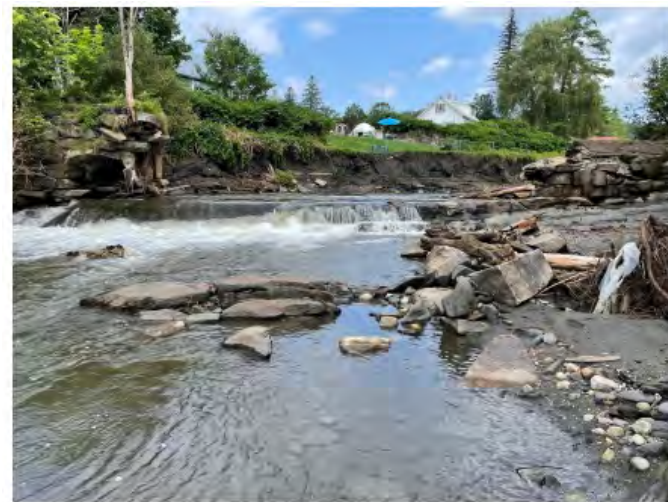
Figure 4: Breached Clark Saw Mill Dam (looking upstream on July 28, 2023)
