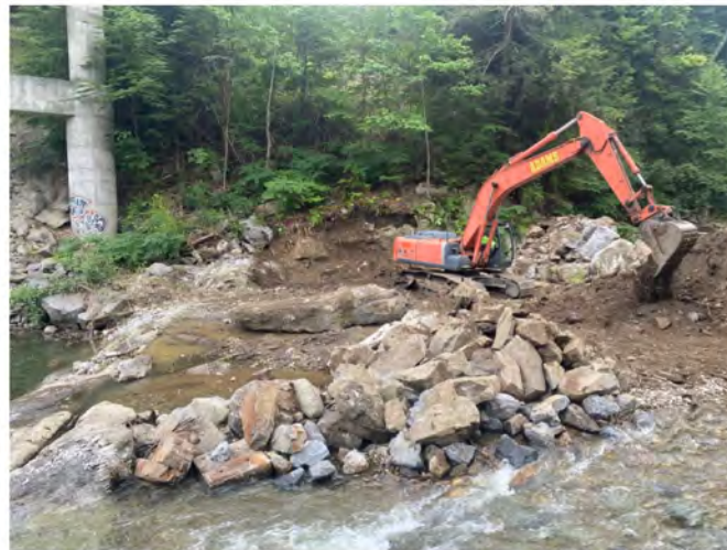
Figure 1: Preparing right bank for stone armor application.
