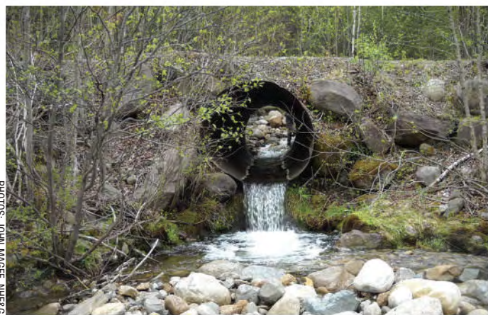
Perched culvert preventing fish movement on Slide Brook, New Hampshire.
