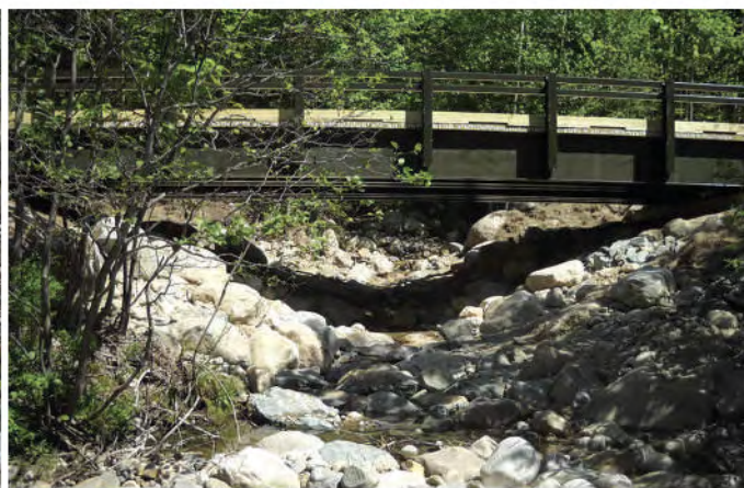
Free-flowing Slide Brook after culvert was removed.
